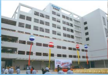
The completed third phase of production facilities.
